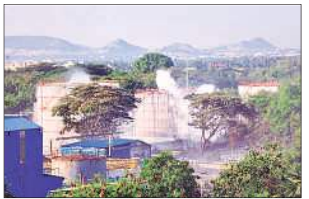
After the gas leak at LG Polymers in RR Venkatapuram village of Visakhapatnam Thursday. P77
