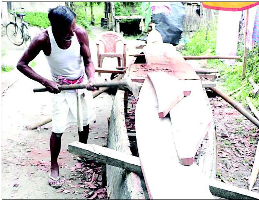
A man repairing a boat ahead of the monsoon in Majuli on Friday. - UB Photos
