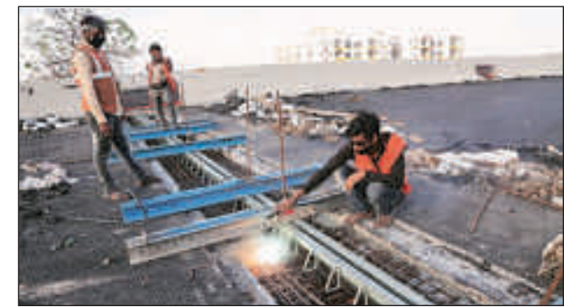
Work on Kharar-Mohali flyover restarted Tuesday. Jasbir Malhi
