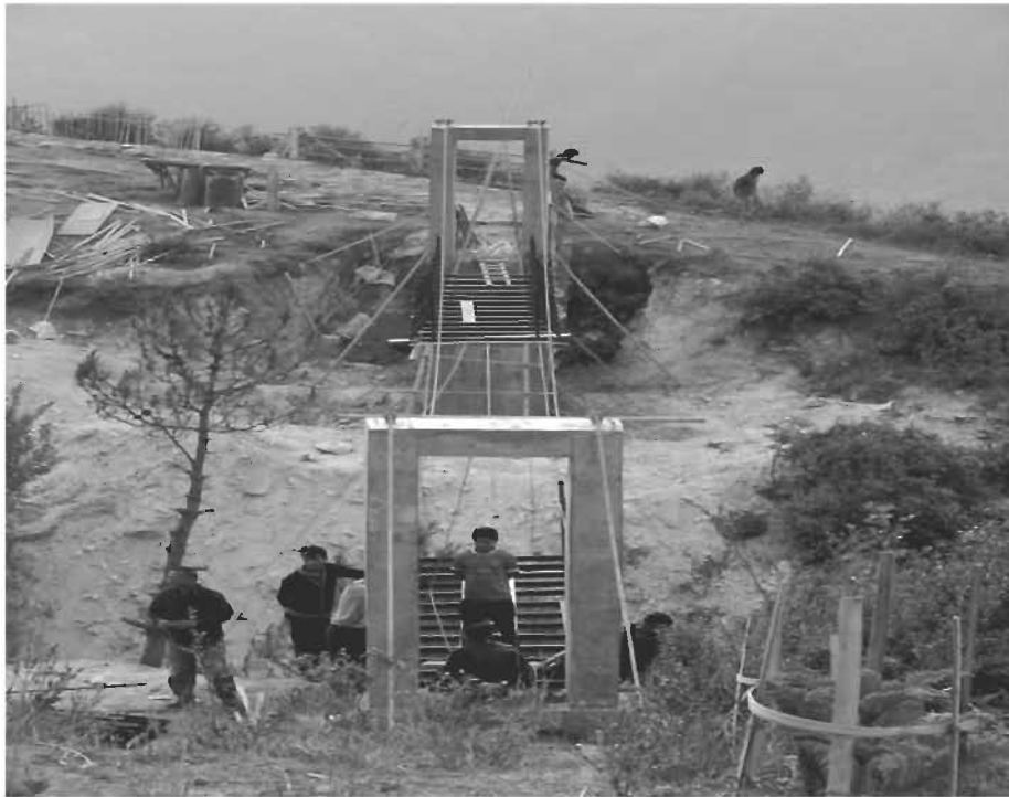
Plate 6: Construction of a new bridge near Heritage Village
